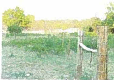
Fence work on west pasture
