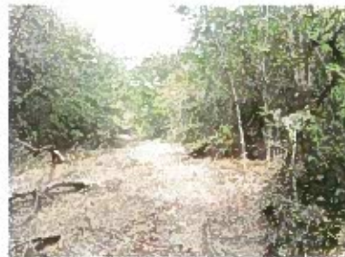
Road clearing in woodland
