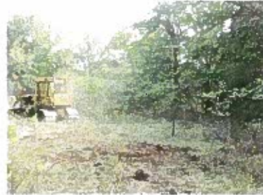
Dozer work on making road
